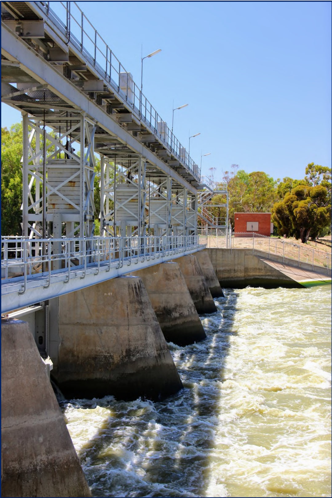
Figure 5. Main Weir, 1 February 2023 releasing ~25,000 ML/d. Source: WaterNSW.
